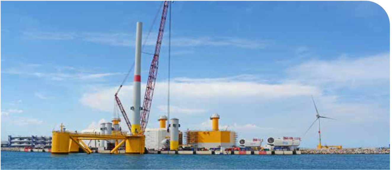
Assembly of wind turbines in Port-la-Nouvelle
