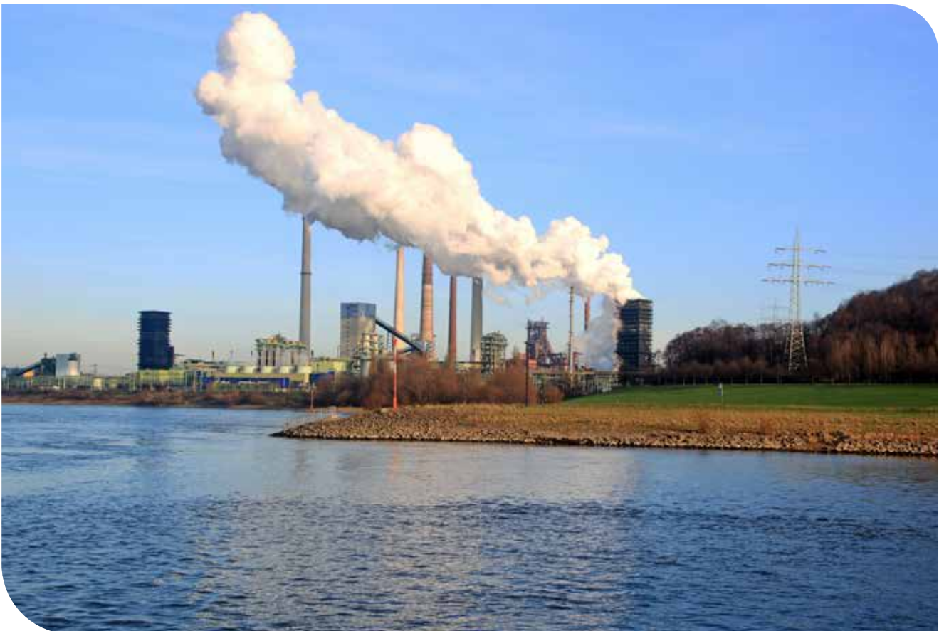
Industrial site in Duisburg (Germany)
