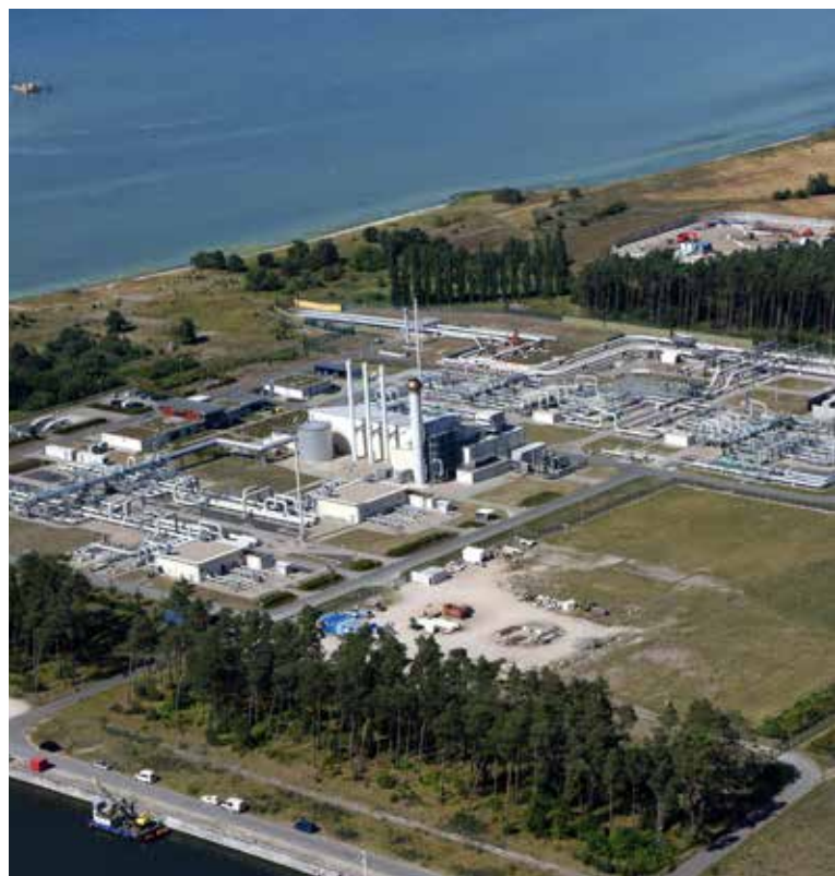
The site at Lubmin in Germany, where the Nord Stream 1 and 2 pipelines come ashore, stands as a symbol of an energy policy long reliant on Russian gas.
